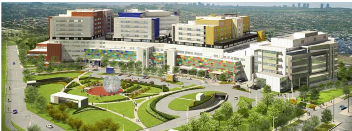
Figure 1 : l'hôpital Royal Victoria du McGill University Health Center (MUHC)
